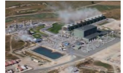
NAP Geothermal power plant
