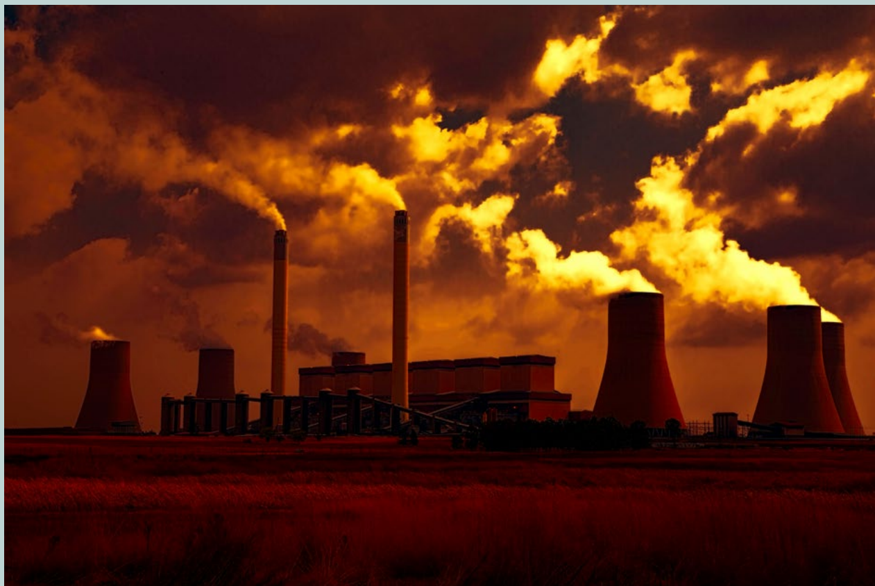
The Drax power station in North Yorkshire, UK, is being modified from coal-fired into a biomass-fired power station. Carbon capture technology is being installed on two of the four biomass-fired generation units. BECCS will enable up to 95 percent of CO 2 emitted during electricity generation to be captured, delivering up to 8 MtCO 2 of negative emissions per year. Storage will be in the North Sea. This project is part of a larger programme to eventually use CCS on all four of its bioenergy units by the mid 2030's.
