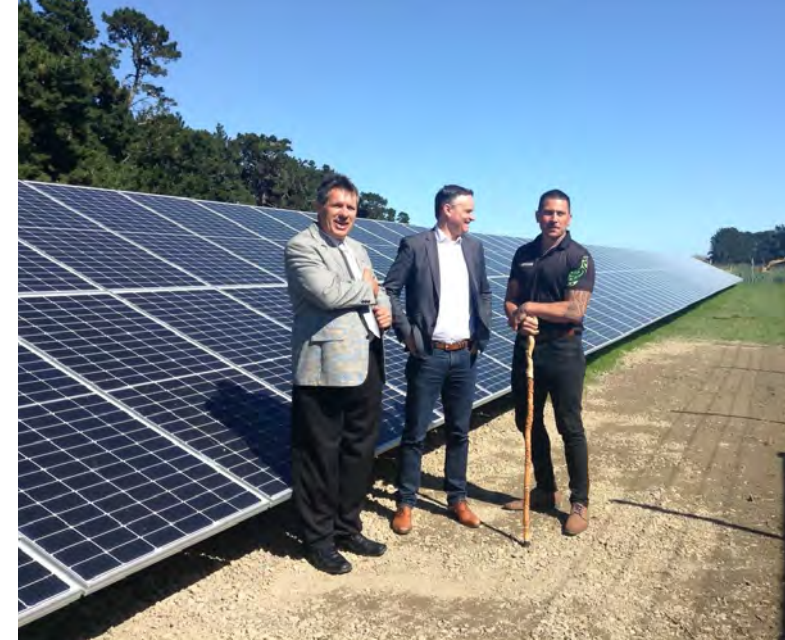
The Rau Kūmara project on opening day
